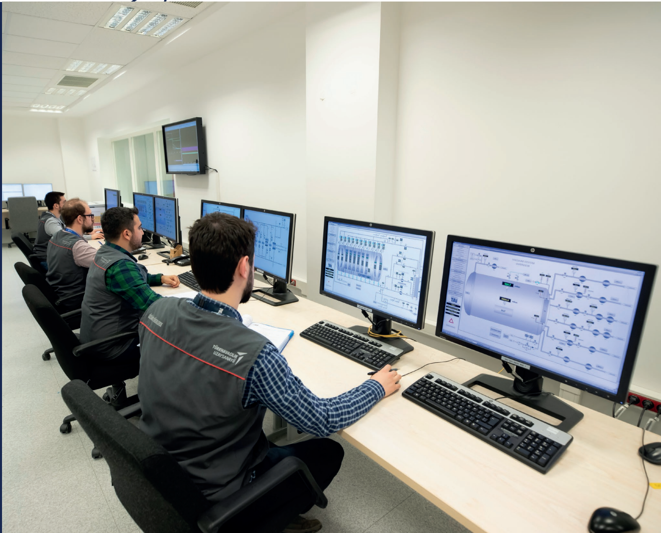
CONTROL ROOM OF TEST SYSTEM
